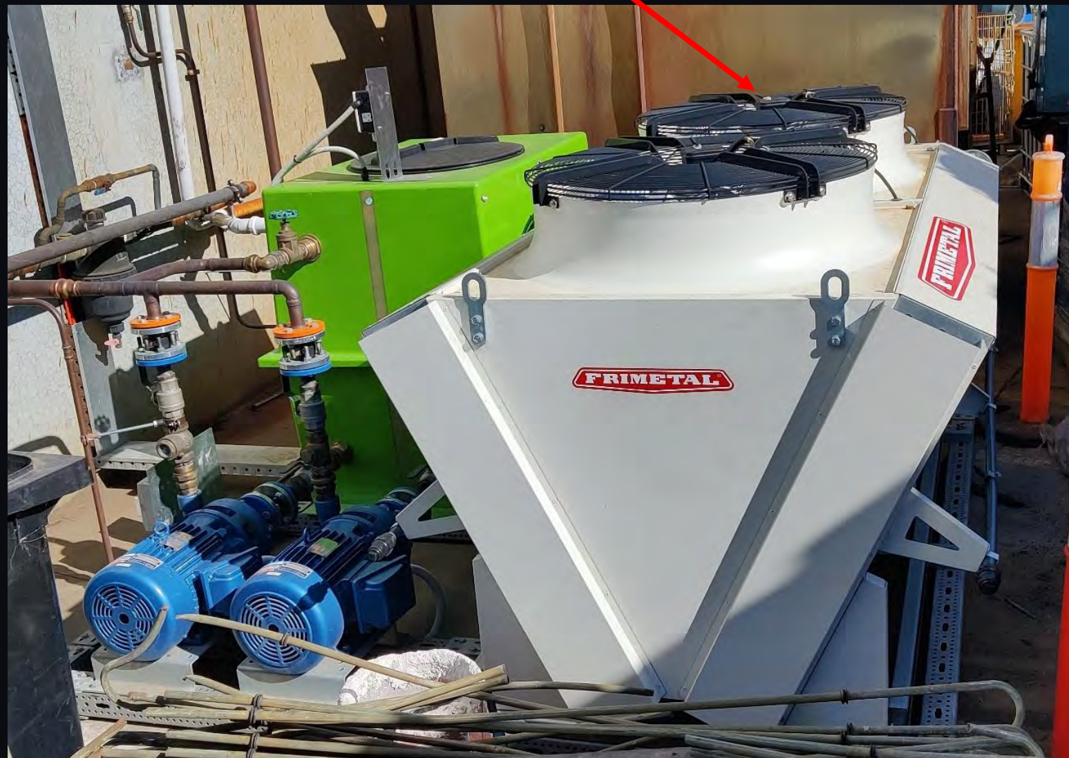
Cooling several Induction furnaces in Melbourne Vic.
